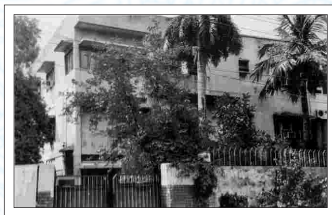
Administrative Block of Kanpur University, Kanpur constructed in 1970s.
